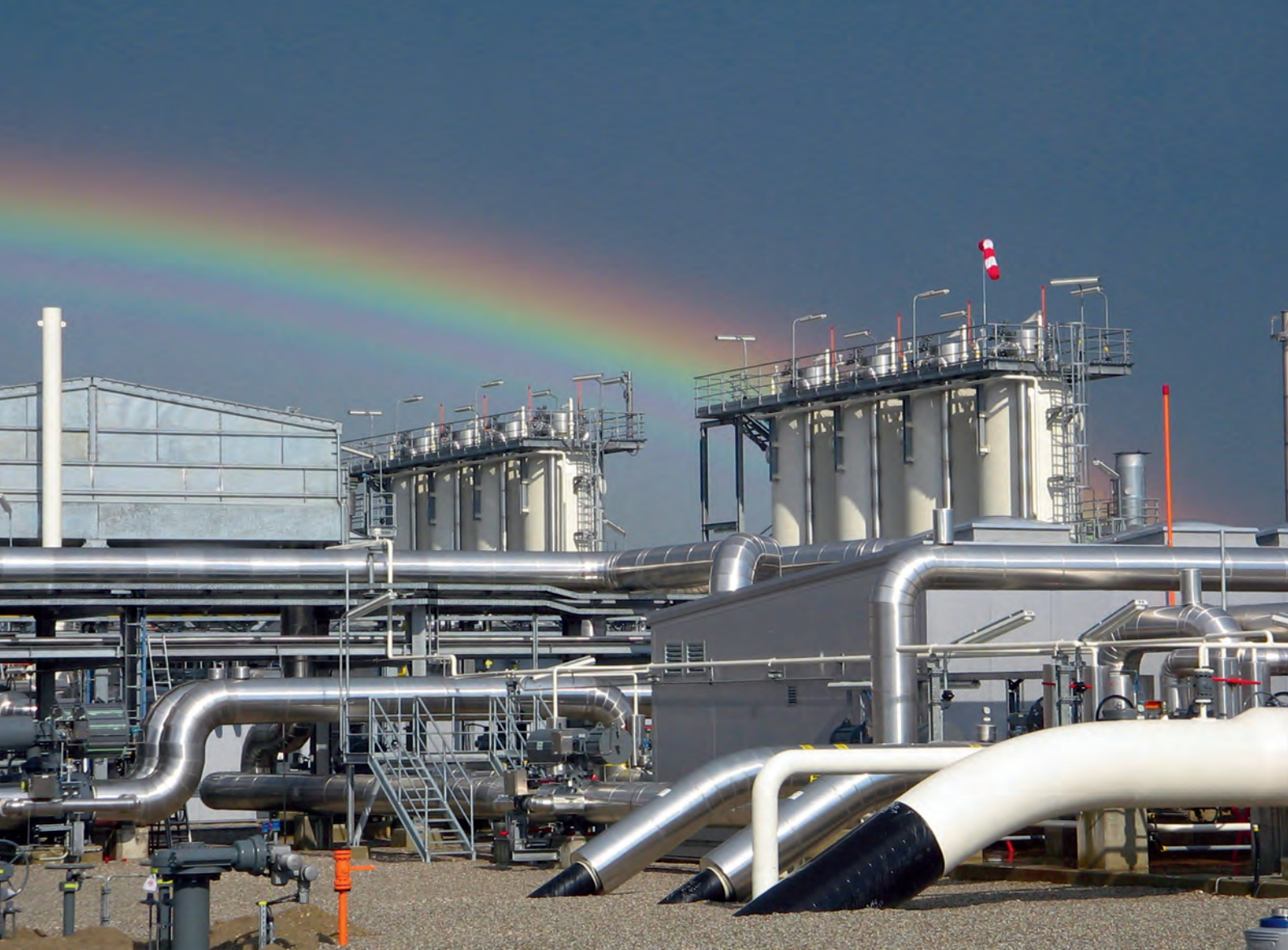
Inlet demister (1) | Adsorber filled with Silica beads (2) Gas-fired heater (3) | Cooler (4) | Outlet dust filter (5)
